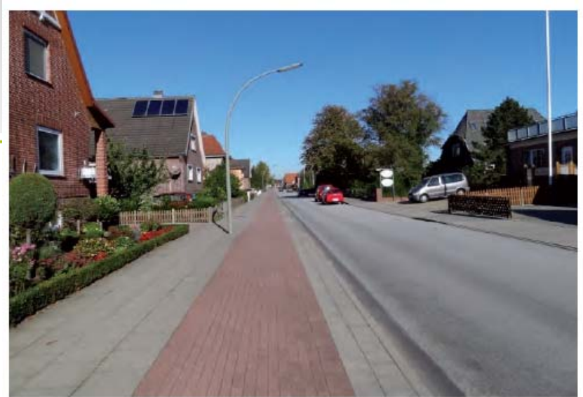
Figure 14: Cycle track in residential area, Hamburg (Germany) Source: Müller 2011
